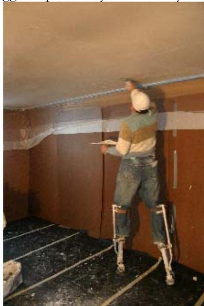
Next they added the sister joists. Finally, they put the ceiling back up. Master plasterer Steve and his assistant Henry replastered the ceiling in two hours. With a fresh coat of paint applied only two weeks after we began, we are ready to show off this restored ceiling when we reopen for tours on Patriots Day.
