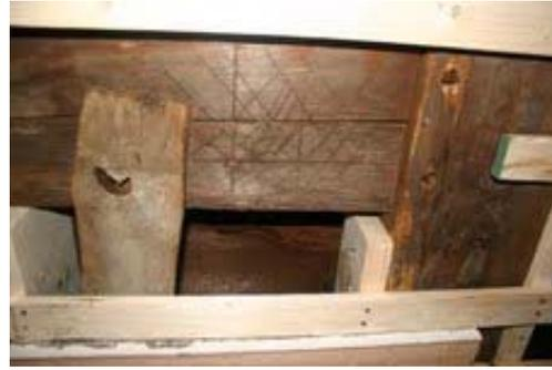
**A view of some of the original Devotion House beams with new support in place.**
