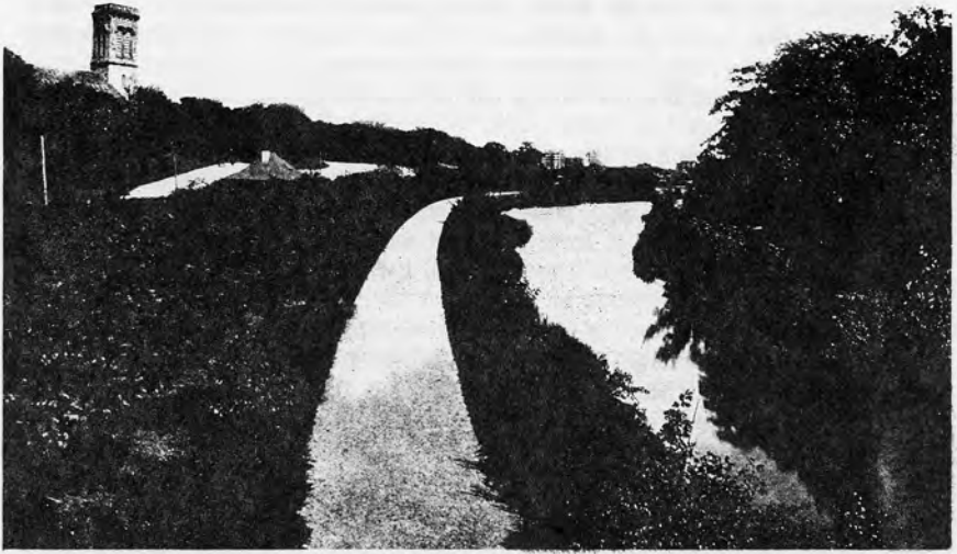
Figure 1 RIVERWAY – VIEW FROM LONGWOOD BRIDGE, LOOKING NORTH
