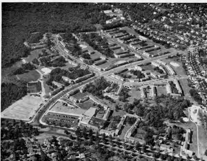
AERIAL VIEW HANCOCK VILLAGE
