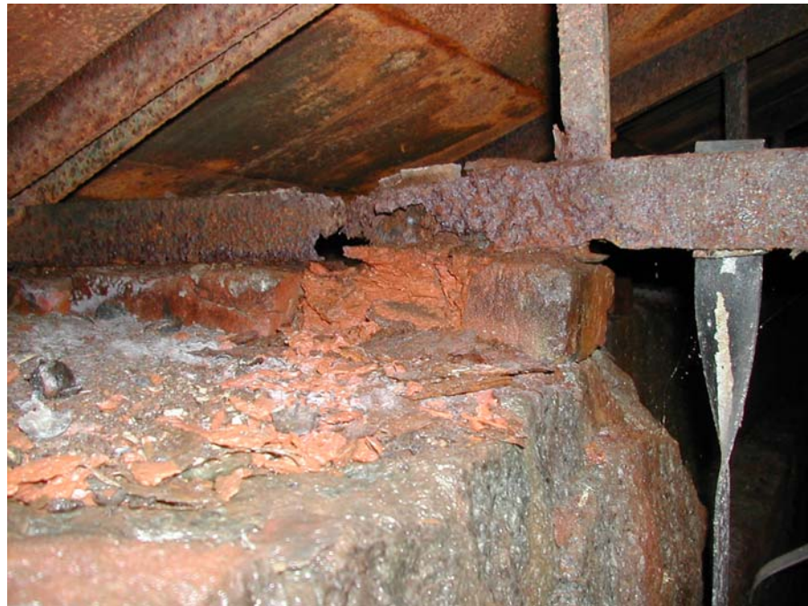
To stabilize and save roof truss ends and clips must be repaired
