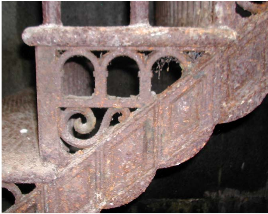
Tread-support of Gatehouse stairs
