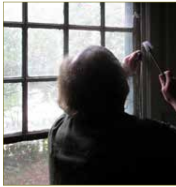
Working on a window.
